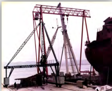
Pile Driving Equipments 7
